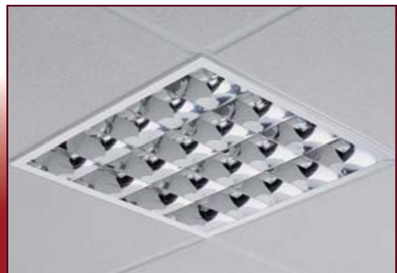
Example of converted emergency light
